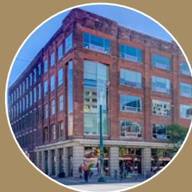
The Robertson Building Toronto, Ontario
